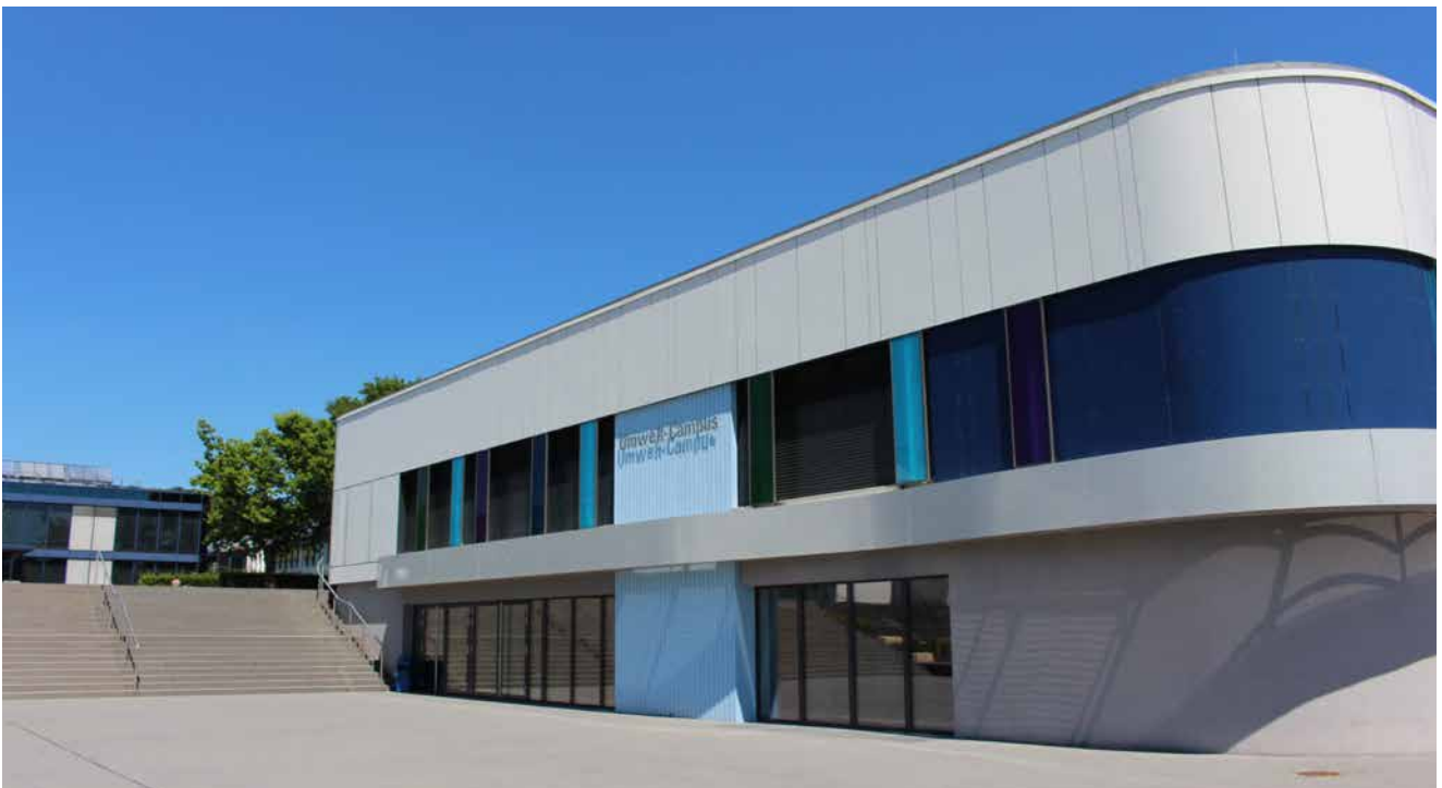
Communications centre at Birkenfeld Environmental Campus.
