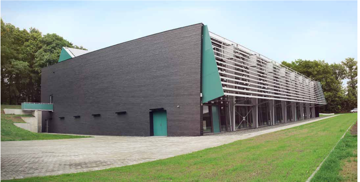
Multifunctional Gymnasium at the Environmental-Campus Birkenfeld
